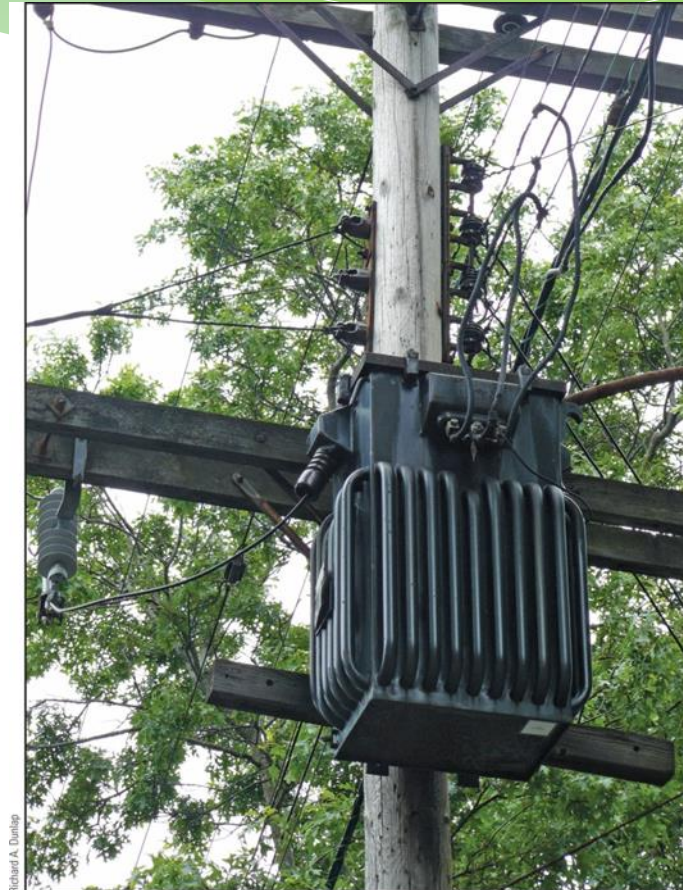
Figure 1.12: Small power distribution transformer on a utility pole in a residential area.
