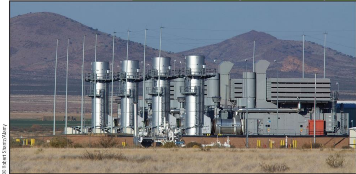
Figure 1.11: Natural gas-fired combustion turbines at the Pyramid Generating Station operated by Tri-State G&T Inc. near Lordsburg, New Mexico.
